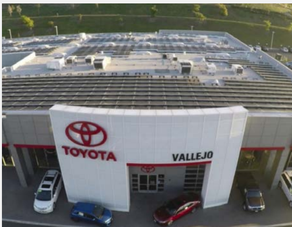
Toyota of Vallejo installed a 251 kW rooftop solar system that is offsetting an average of 61 percent of the dealership's electricity needs.
